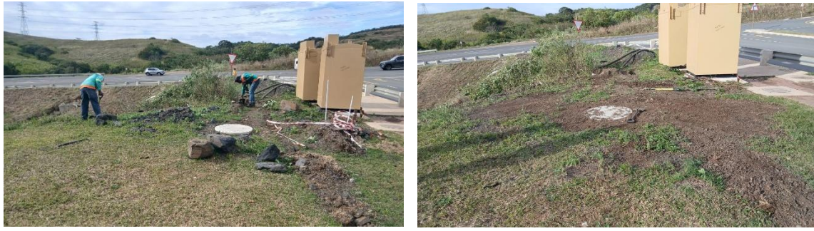
Photos above - maintenance work done by Idube Landscaping
